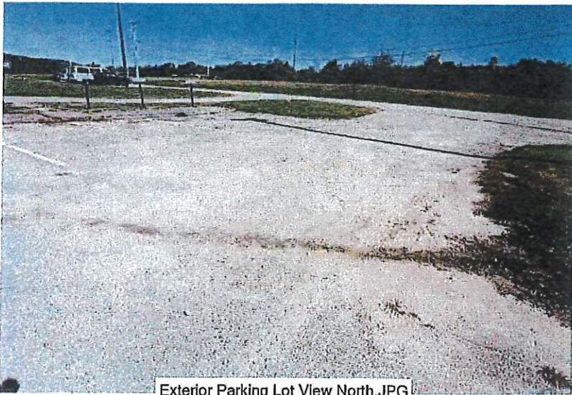
Exterior Parking Lot View North.JPG
